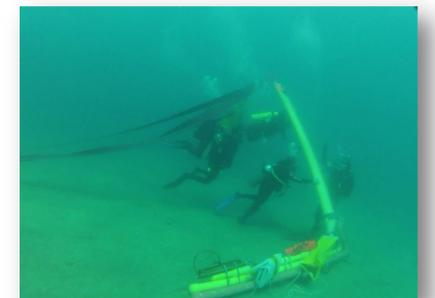
After 3 successful deployments, it was confirmed that fluidization is a viable method of burial and sand management. The Fluidizer was able to bury itself to a depth of 2 ft. At this depth, it was also able to fluidize and remove the sand, leaving a trench of absent material behind.
